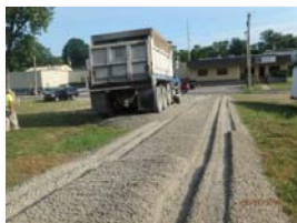
Paving trailer lot with gravel
